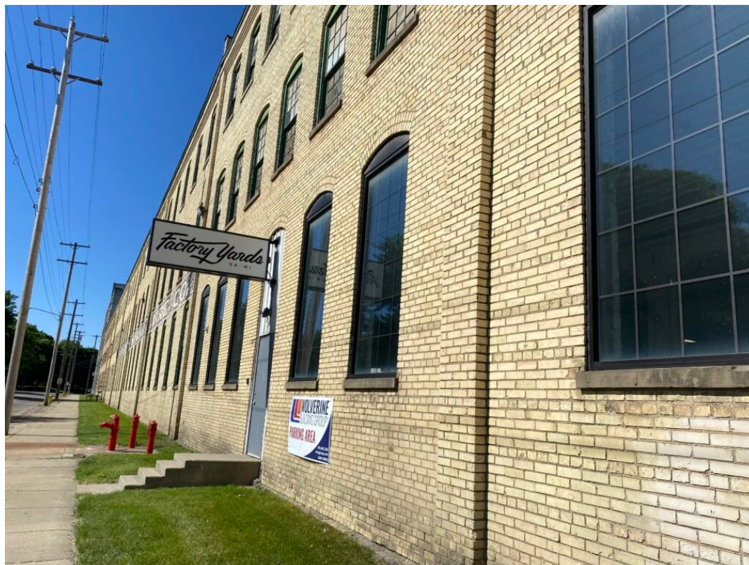
Heritage Development has started work on the $147 million mixed-use Factory Yards project, a renovation of a long-vacant 15.5-acre industrial property near 655 Godfrey Ave. SW. Credit: Kate Carlson, Crain's Grand Rapids Business
